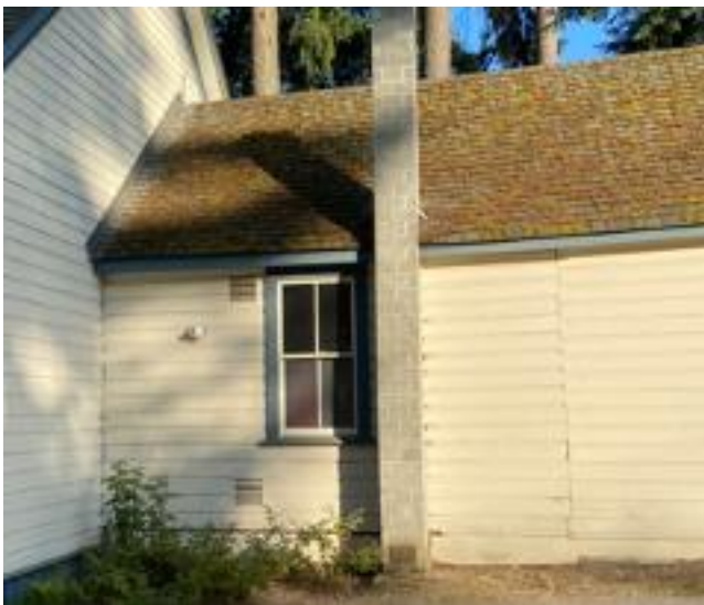
Change in siding showing the extent of the original classroom
