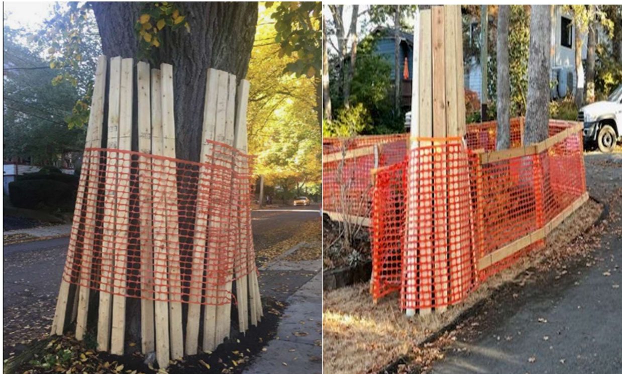
Figure 8- Tree Protection and Signage
