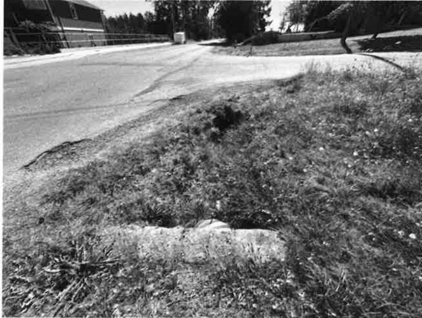
Photo 1. Roadside ditch and culvert at the eastern property extent, looking south (downstream). September 7, 2022.
