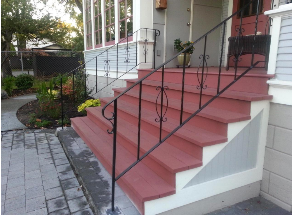
Duplicating wrought iron railing so home can remain heritage status
