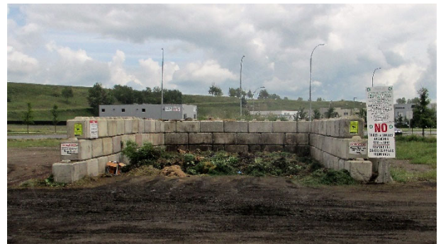
Figure 11-2: Example of Bunker for Yard Waste
