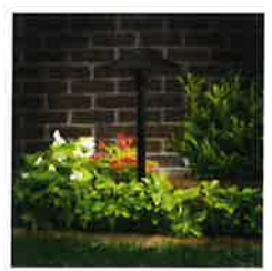
6 Downcast landscape lighting
