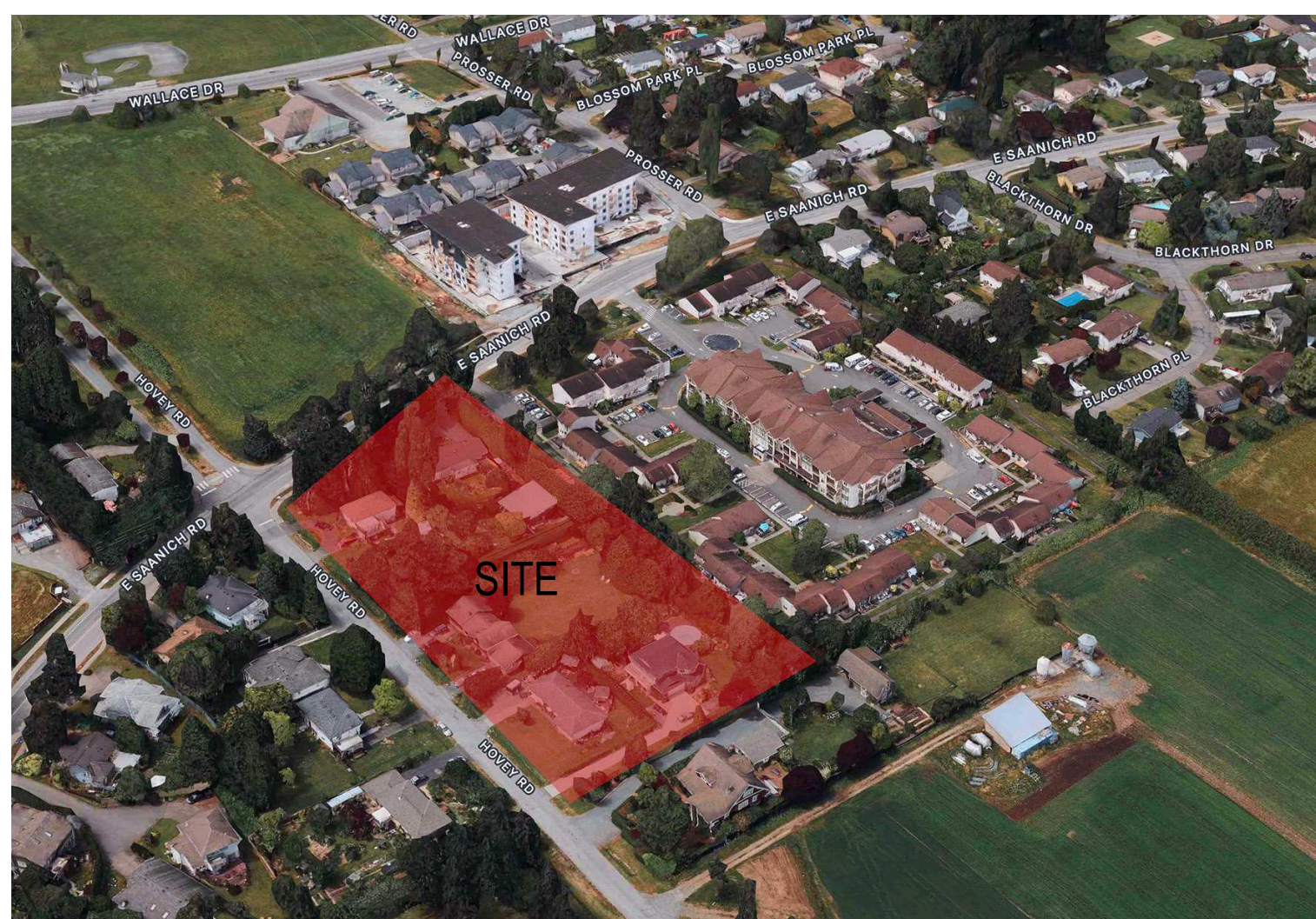
DRONE VIEW - LOOKING NORTHWEST
