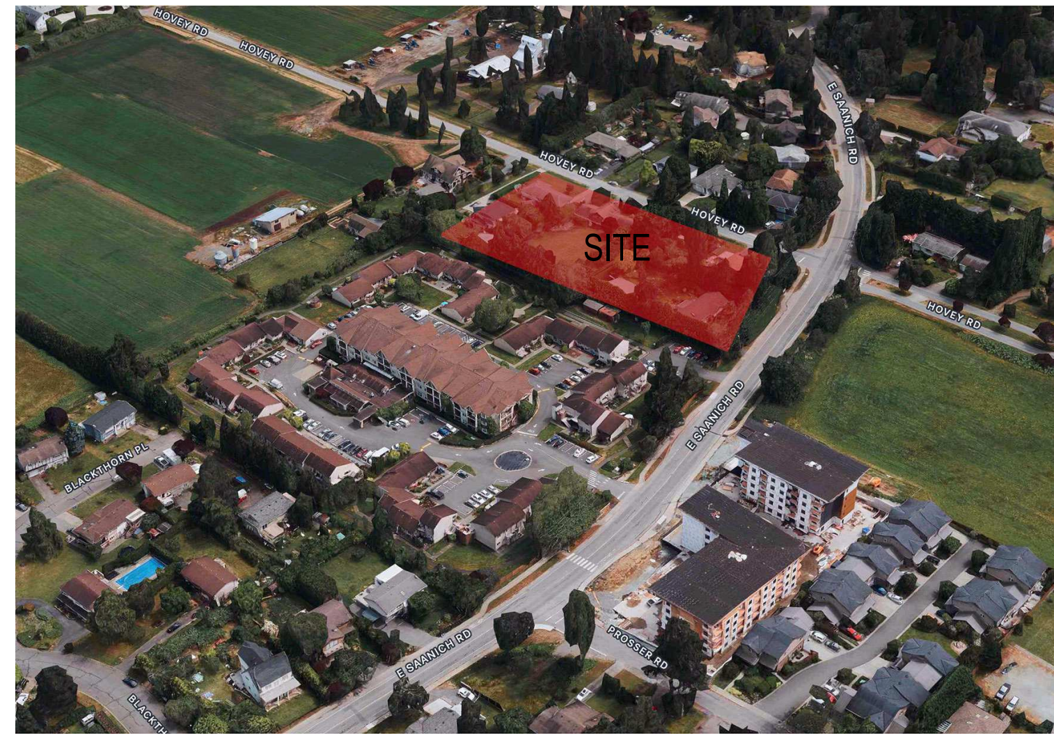
DRONE VIEW - LOOKING SOUTHEAST
