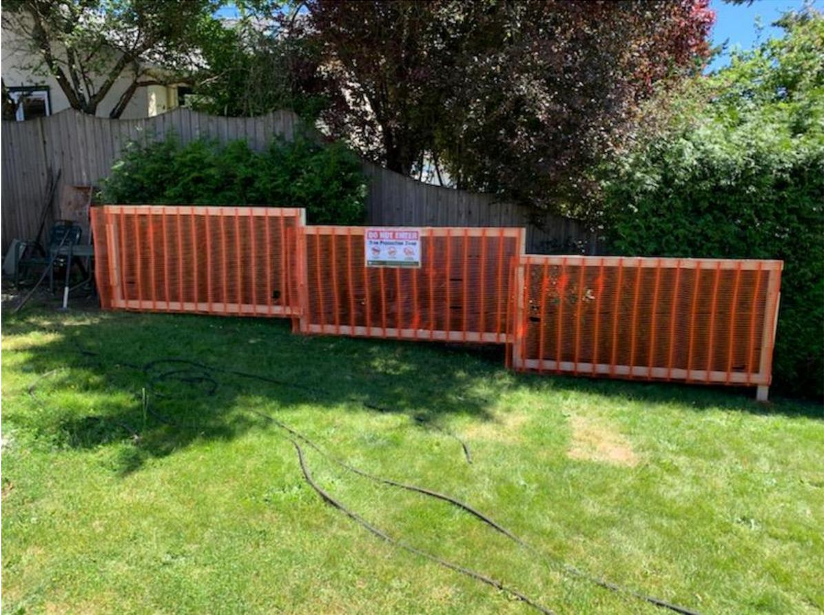
In this photo you can see the basic design and construction requirements for Tree Protection Fencing in the District of Central Saanich. The sign on the front of the fencing is required. The sign must be posted in a visible position on the fencing.
