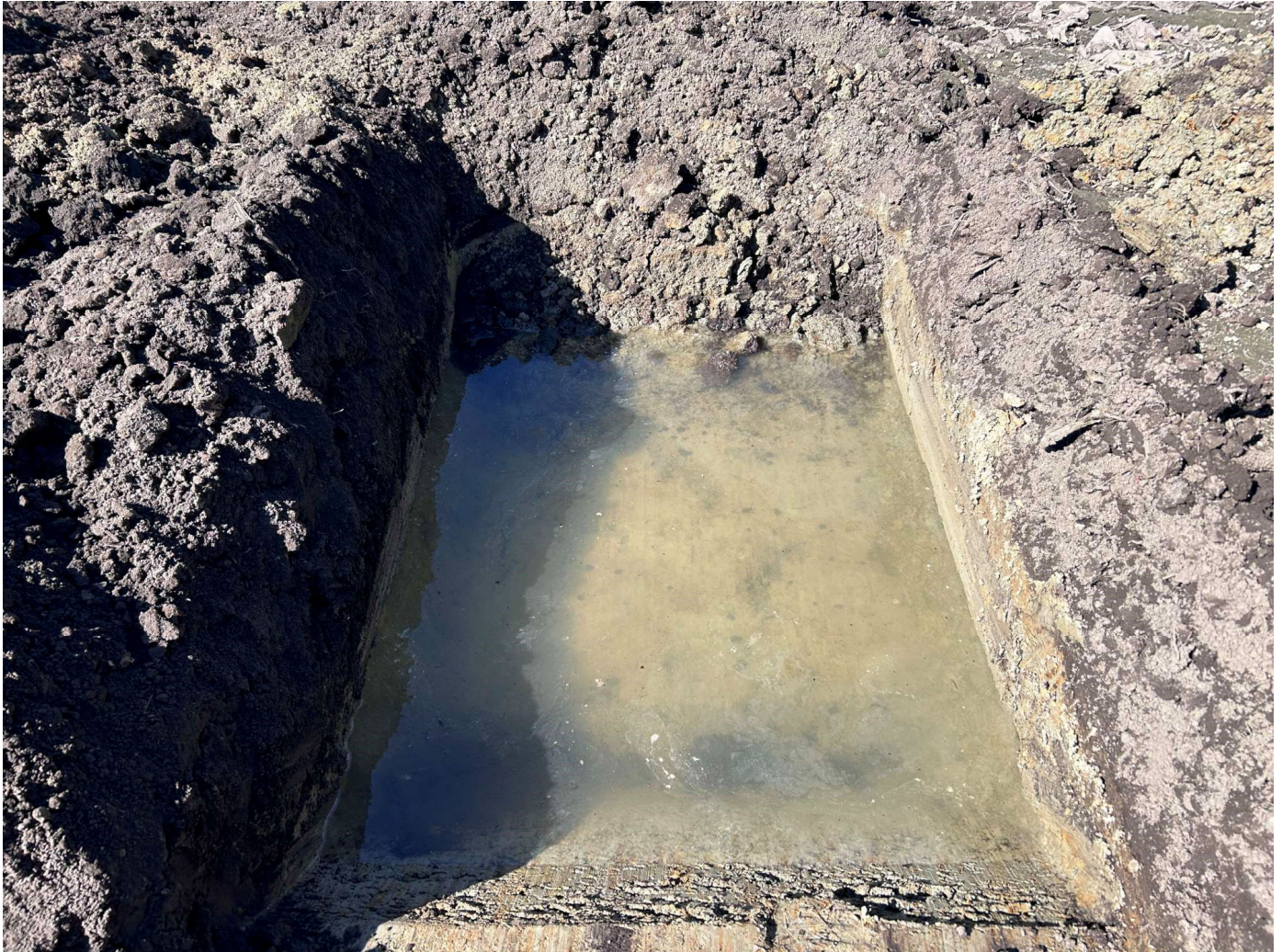
Typical shallow test pit into native clay with ponded water
