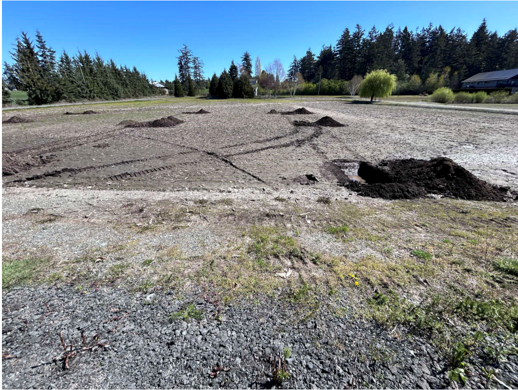
Southern portion of area looking east from southwest corner
