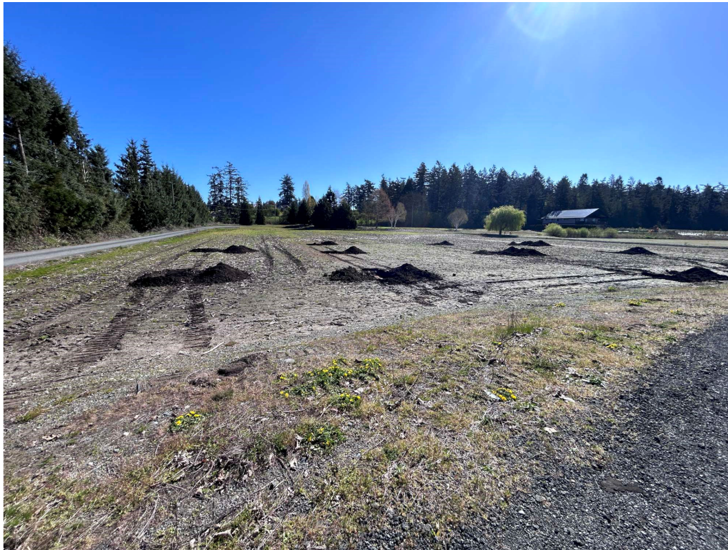
Northern portion of area looking east from northwest corner
