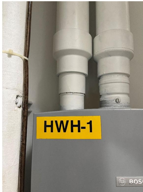
Figure 8: DHW Gas-Fired Water Heater (Upper Mechanical Room)
