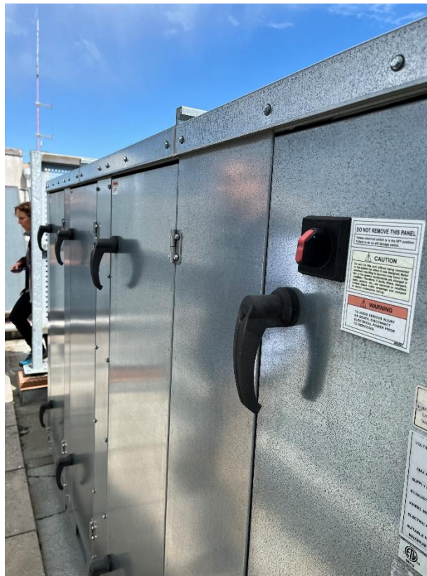
Figure 5: Heat Recovery Ventilator (Rooftop)
