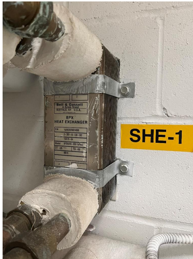
Figure 10: Solar Thermal Collector Heat Exchanger (Upper Mechanical Room)
