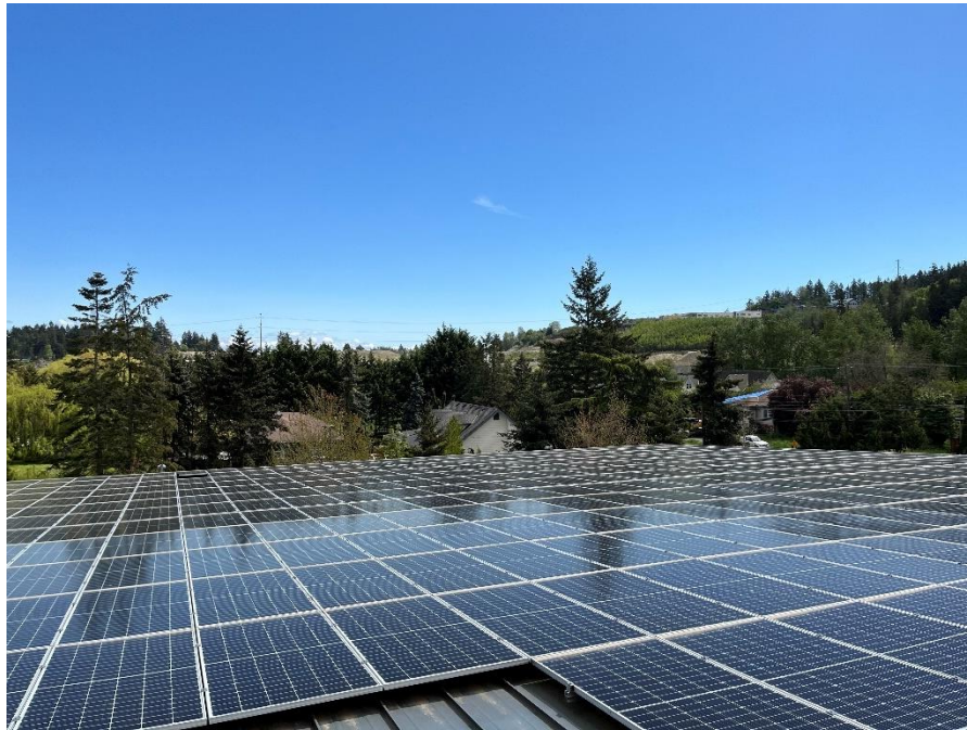
Figure 11: PV Array, 138kW (Rooftop)
