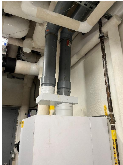
Figure 3: Heating Plant Gas-Fired Boiler (Lower Mechanical Room)
