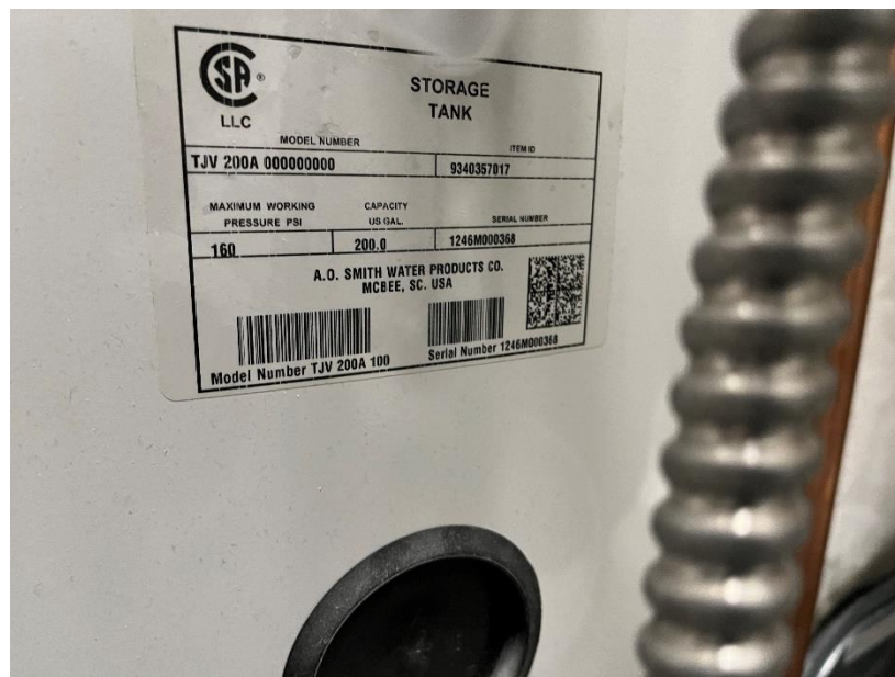
Figure 7: DHW Storage Tank Nameplate (Upper Mechanical Room)
