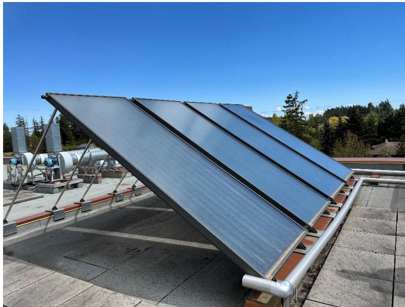
Figure 9: Solar Thermal Collectors (Rooftop)
