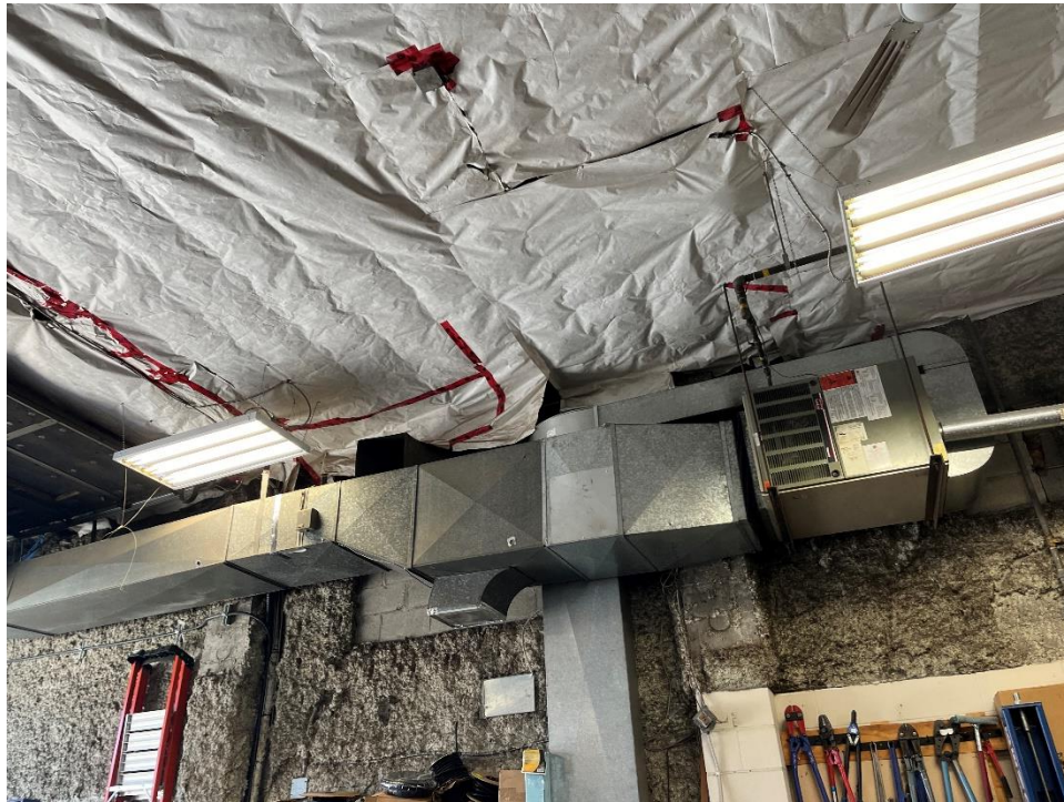
Figure 1: Main Building Gas-Fired Air Handling Unit
