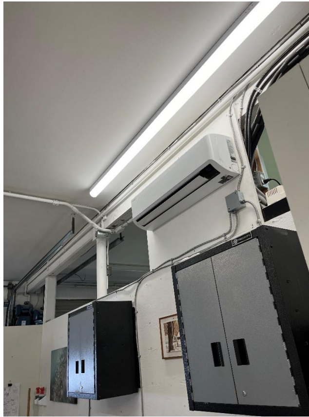
Figure 5: Locker Room Wall-Mounted Cassette
