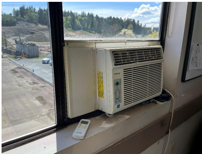
Figure 4: Upper Office "Window-Shaker" Condensing Unit
