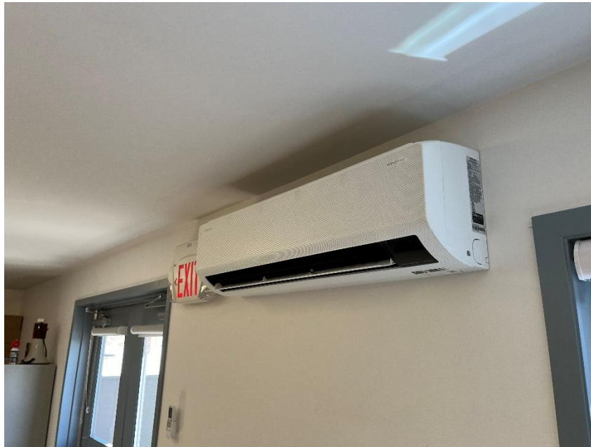
Figure 3: Common Space Wall-Mounted Cassette
