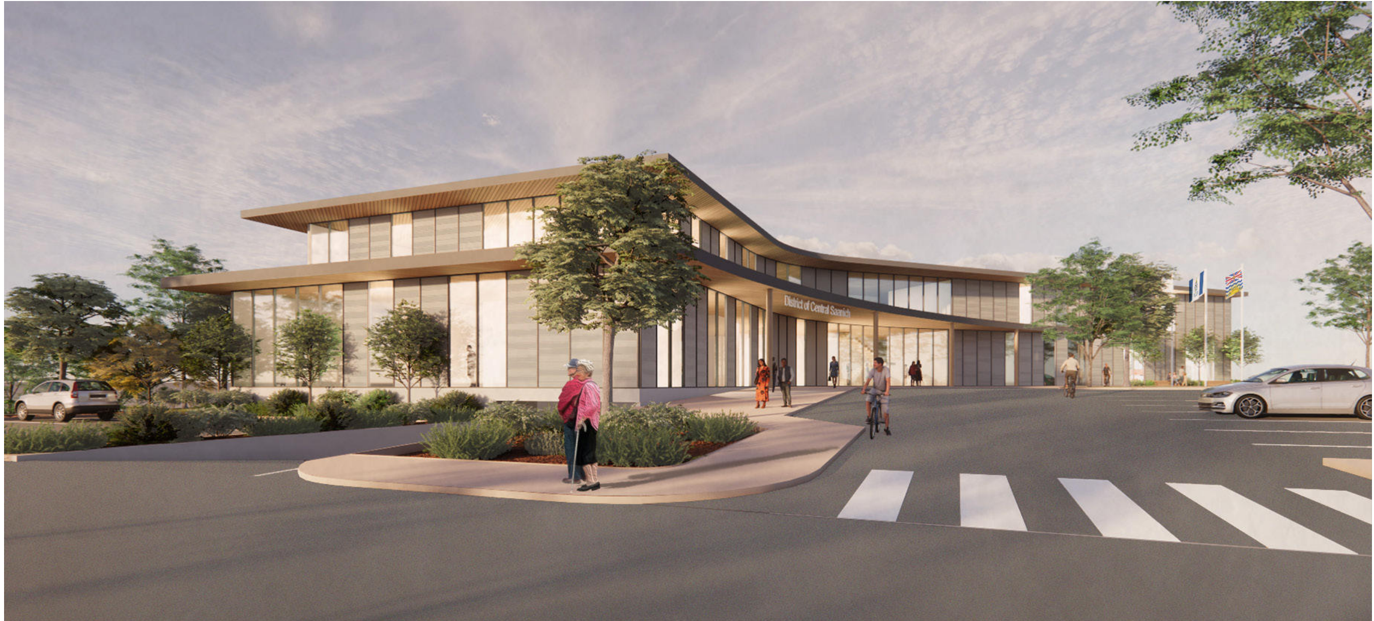
View of Entrance from South of Site
